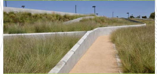
Terraced Retaining Walls
