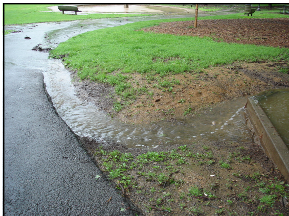
75. Stream of water from overflow at catch basin, west entrance of tunnel
