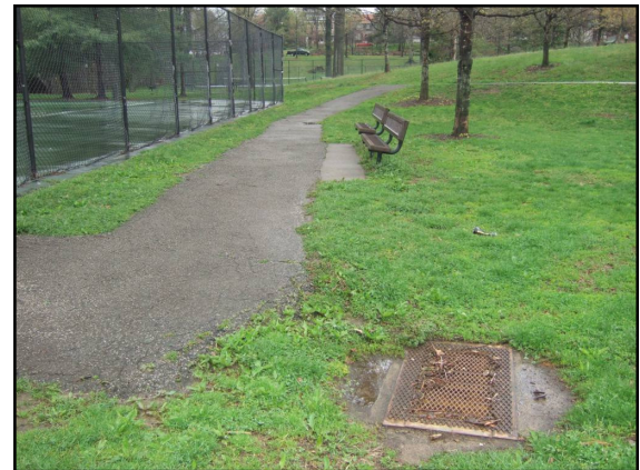
30. Catch basin near south tennis courts
