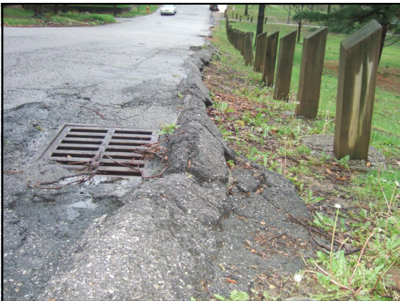
11. Catch basin along Tyler Park Drive, looking southeast
