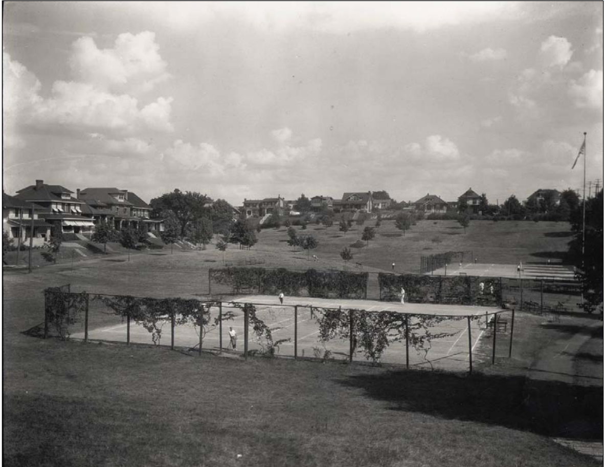
Figure 2: The size of trees and other plantings in this undated view southeast from the northwest corner of Unit 2 at Baxter Avenue suggests that it was taken at a later date than Figure 1. Vines stretch across the wire fence of the tennis courts. Single trees are scattered on the sloping south hillside, opposite the camera. In this photograph, park visitors use the tennis courts for active recreation, a use accommodated by the Olmsted Brothers' 1907 design. Courtesy Metro Parks. (R-THL-MP-Tyler-Undated.jpg)
