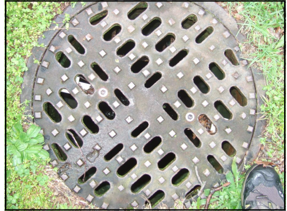
28. Closeup of combined sewer manhole
