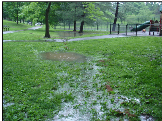
72. Standing water at catch basin between south tennis courts and tunnel
