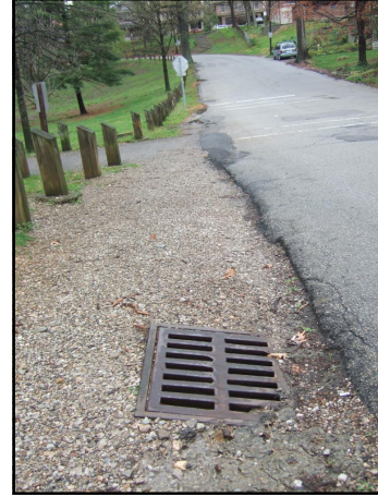
20. Catch basin in gravel shoulder along Tyler Park Drive
