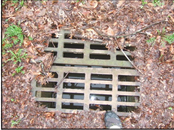
49. Closeup of catch basin
