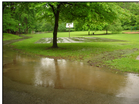
76. Poned water on walkway in front of bathrooms
