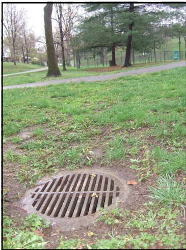
33. Catch basin between south tennis courts and tunnel
