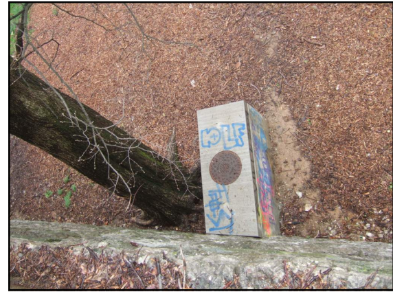
60. View of above-grade manhole box, from Baxter Ave.
