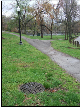
27. Combined sewer manhole at southeast corner of park
