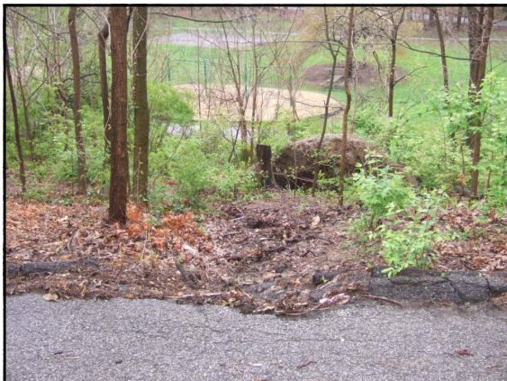
53. Erosion of slope, from Tyler Park Drive runoff
