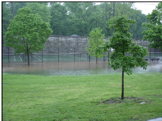
71. Severe ponding east of the south tennis courts
