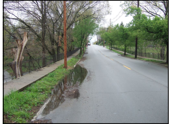
62. Standing water on southwest side of Baxter Ave.
