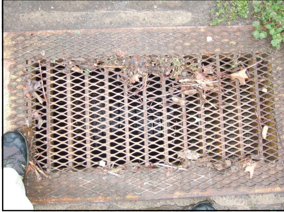
31. Closeup of catch basin
