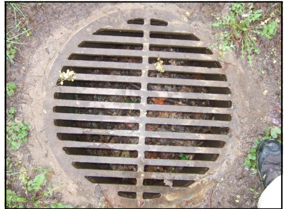
34. Closeup of catch basin
