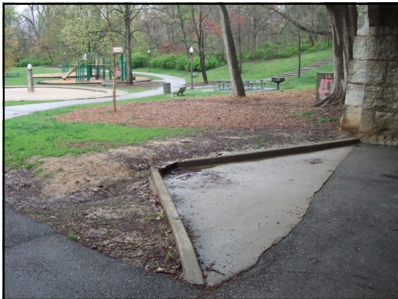
39. Catch basin at west entrance to tunnel
