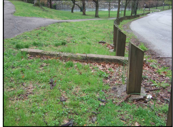
26. Concrete headwall near southeast corner of park
