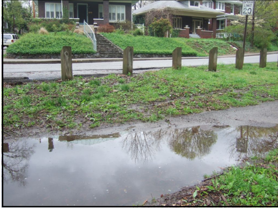
25. Standing water near lightpole
