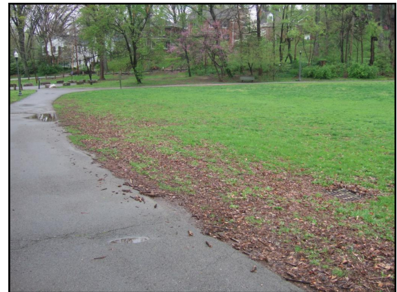
48. Standing water on sidewalk, catch basin to the right
